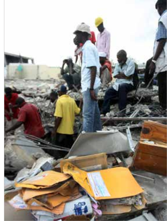
The 2010 earthquake in Haiti left post offices destroyed.
