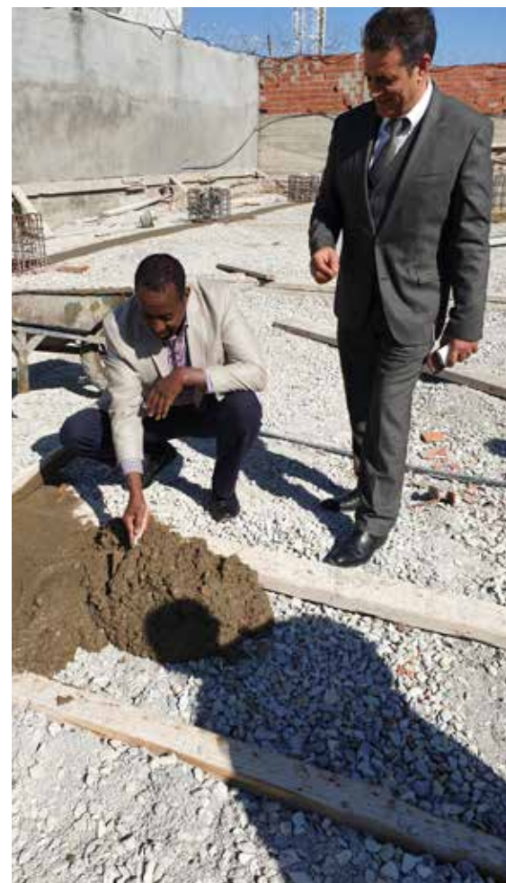
The UPU Director General Bishar A. Hussein sets the first foundation at the Tunis Ecom@Africa fulfilment centre.
